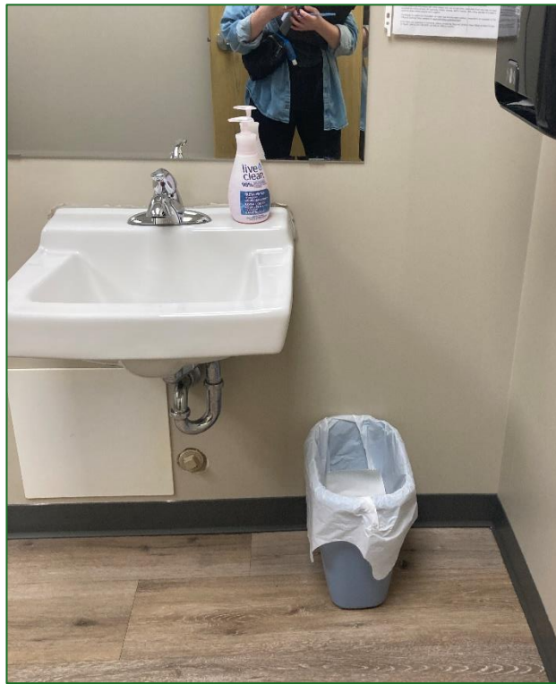
Figure 16 The pipe under the sink in the accessible washroom is uninsulated.
