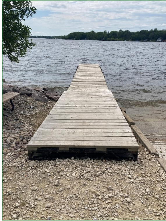
Figure 29 The dock at the Fernwood Boat Launch is long and would benefit from a railing. It also has a step up between the dock and the ground that could be addressed with a transition ramp.
