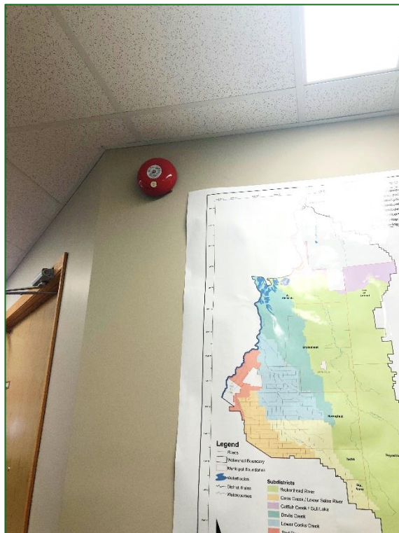
Figure 13 The fire alarm system at the municipal office does not appear to have visual/light components.
