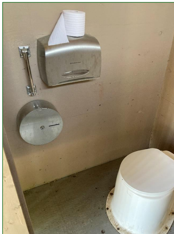
Figure 41 Towel bars are being used as grab bars at the Halliday Park washrooms. They are installed behind the toilet paper dispensers, so they are out of reach of anyone who needs them.
