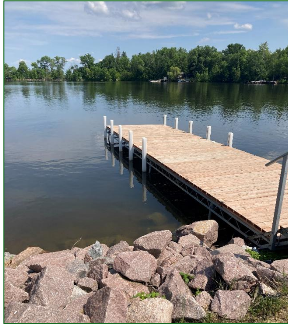
Figure 27 The railing on the stairs at the Winnipeg River Boat Launch could be continued onto the dock.
