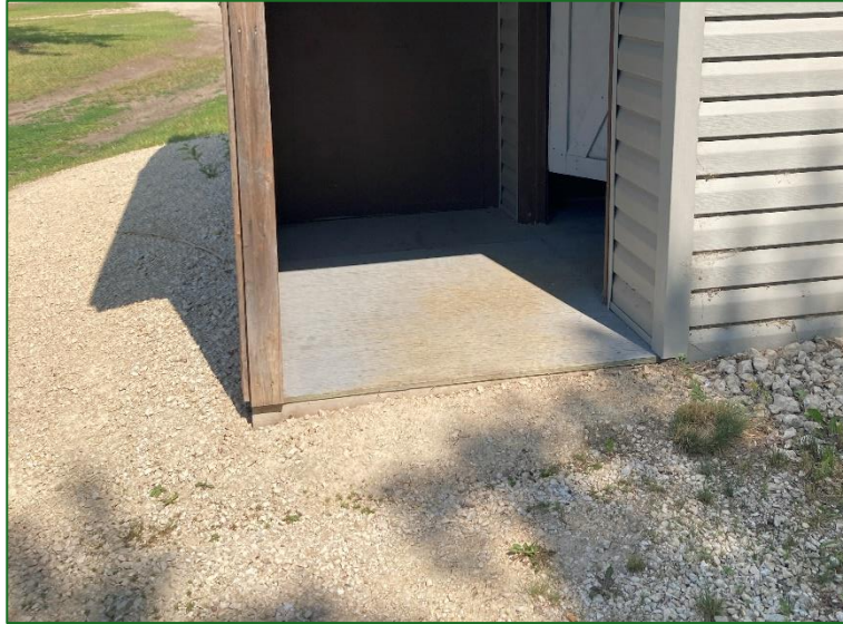
Figure 44 The entrance to the public washrooms at the LaVerendrye site. There is a lip between the edge of the platform and the gravel underneath that creates a barrier for people using mobility aids.
