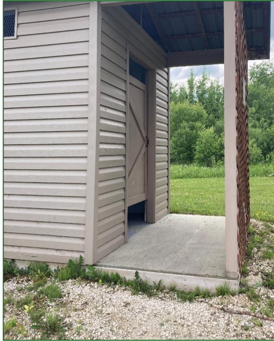
Figure 46 The path leading to the Lac du Bonnet Trout Ponds washroom is uneven and there is a step up onto the washroom platform.
