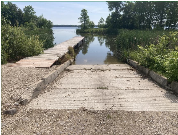
Figure 20 The gravel leading up to the dock at the Wood Duck Boat Launch is uneven at the edge of and leading up to the dock. The concrete edge on the boat launch ramp has also broken and worn away.
