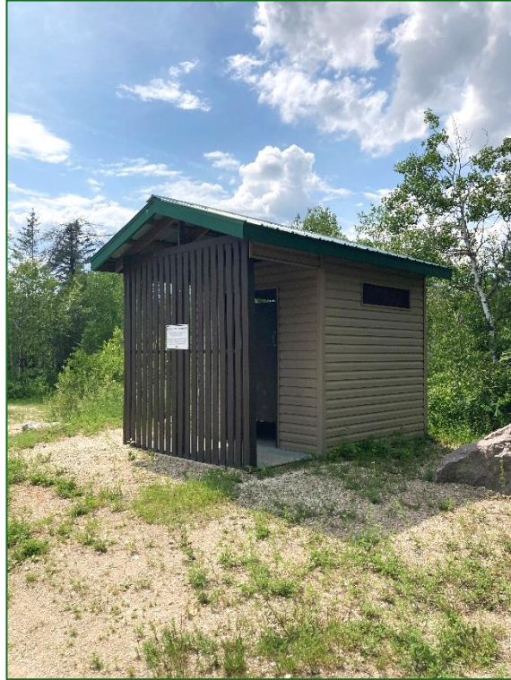
Figure 47 The washroom at the Blueberry Rock Trail is located on an incline. The path leading up to the washroom is also uneven and weeds are growing through the gravel. There is also a step up from the gravel to the washroom platform.
