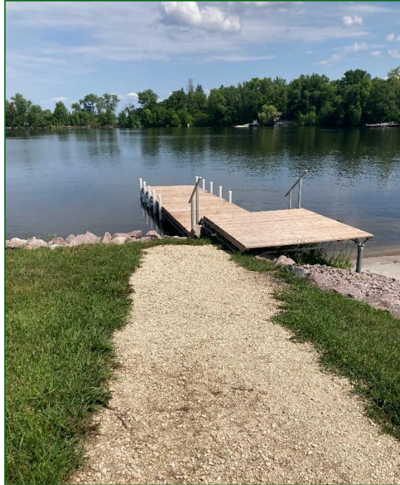
Figure 24 There is a step up between the path and the platform leading to the dock at the Winnipeg River boat launch.
