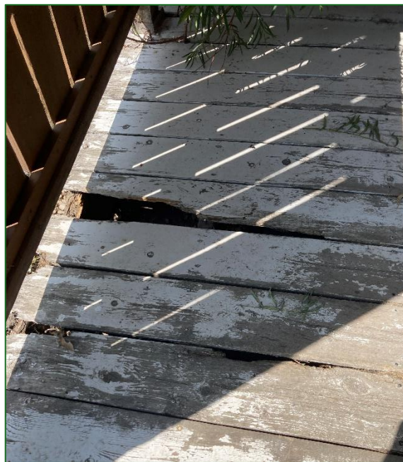
Figure 45 The platform at the Winnipeg River Boat Launch public washroom is decaying and poses a tripping hazard.
