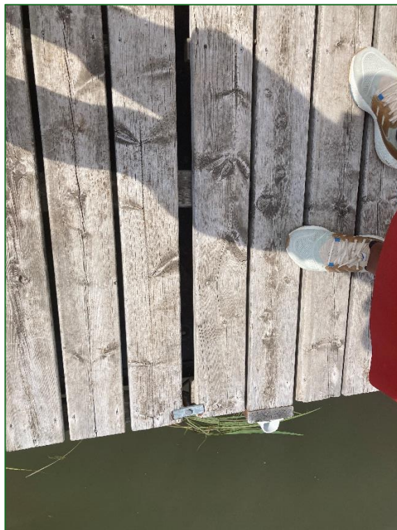
Figure 25 There is a gap in the boards on the dock at the Wood Duck boat launch site.
