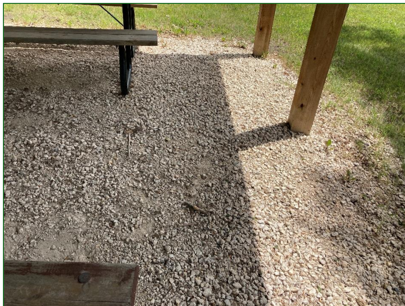
Figure 54 The gravel under the picnic area at Fernwood Park is mostly even, but it appears to have loosened due to weather and foot traffic.
