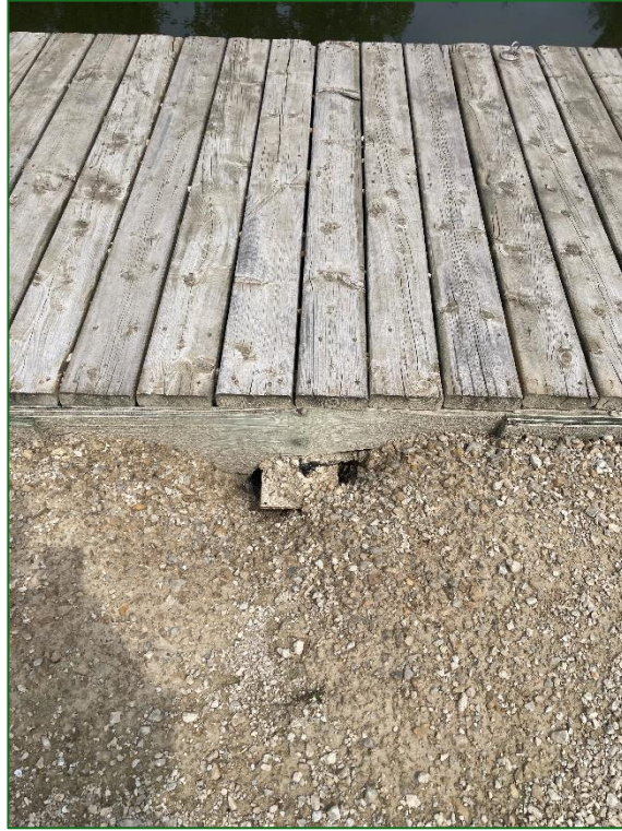
Figure 19 At the Osprey Boat Launch, there is a tripping hazard where the gravel has worn away at the dock.
