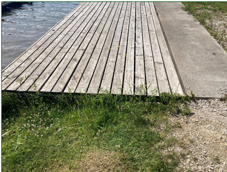
Figure 22 The dock at the LaVerendrye boat launch has foliage growing close to the edge. The gravel path leading to the dock is also uneven, and the gap between the dock and the ground is a tripping hazard.
