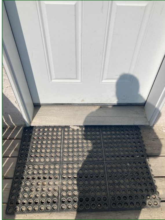
Figure 9 The threshold of the door at the public works office could present a tripping hazard.
