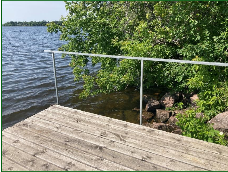
Figure 30 The dock at the LaVerendrye boat launch has a railing, but the railing does not have cross bars.
