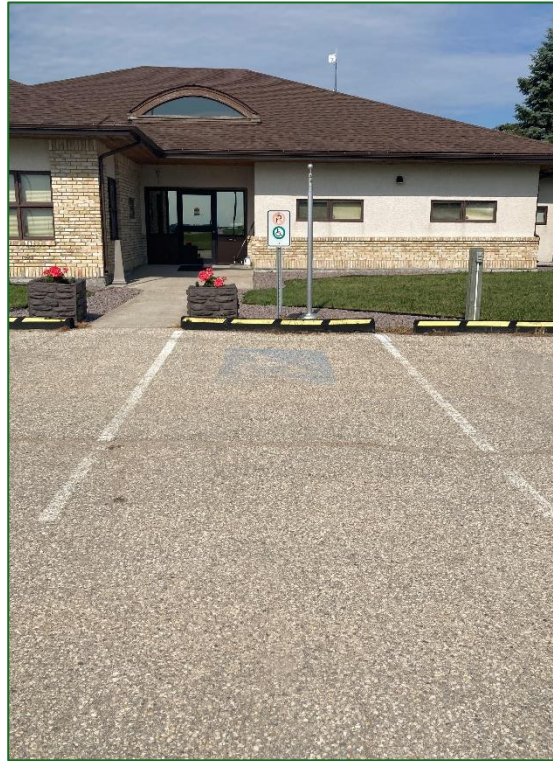
Figure 6 The painted sign denoting the accessible parking space is very worn. While the sign is still in good condition, refreshing the paint would provide another important visual cue about the space.
