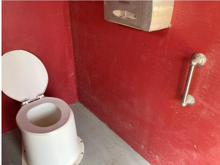
Figure 40 The Osprey Boat Launch washrooms appear to have towel bars installed instead of actual grab bars. The grab bars are also installed far from the toilets, out of the reach of many people.
