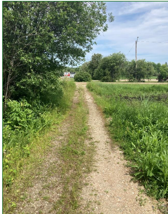
Figure 51 Grass and foliage growing into the surface of part of the Cape Coppermine Road trail makes the space on the trail narrower.
