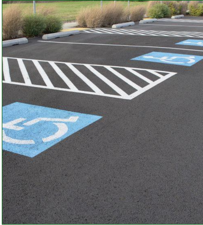
Figure 7 An example of effective parking lot paint design, with diagonal line striping across the walkway between two accessible spaces. From the UrbanPaint.ca website.
