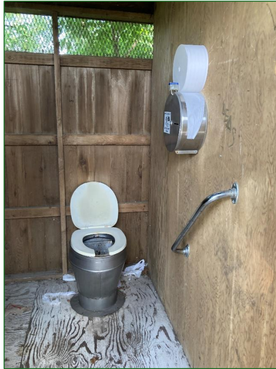
Figure 42 The toilet dispensers in the Winnipeg River Boat Launch washrooms are installed high on the walls, outside of the reach of many people when seated on the toilet.
