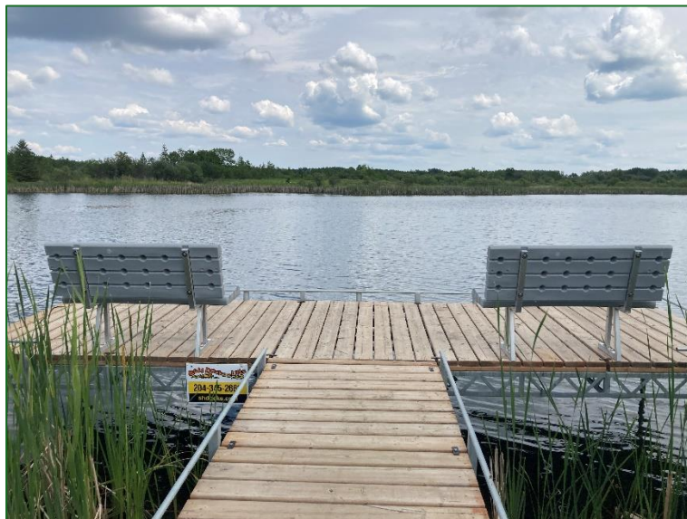
Figure 28 The dock at the Lac du Bonnet Trout Ponds would benefit from a railing behind the benches to prevent falls.
